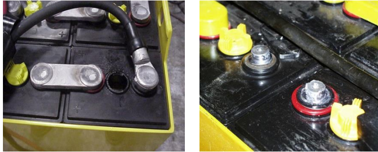
Figure 7: Remove the last intercell connector and clean the posts
